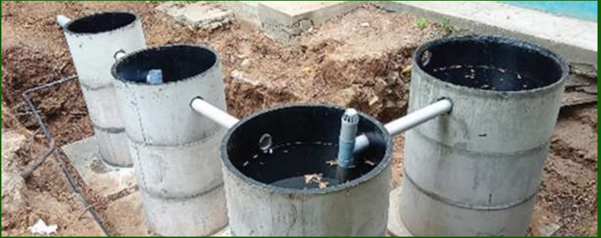
Textile-reinforced concrete precast units.
