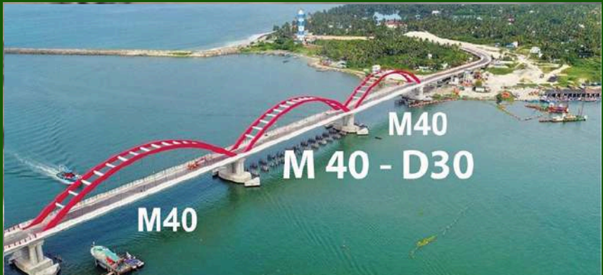
Slag-based concrete for extending service life and reducing the carbon footprint of a coastal highway bridge.
