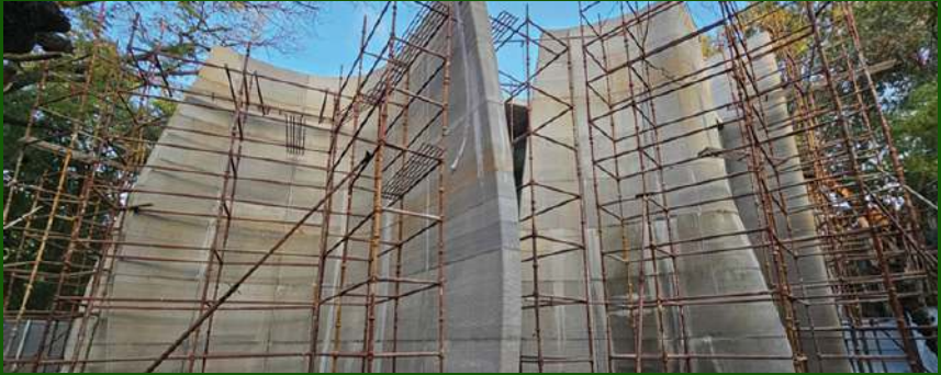
Construction of a G+1 3D-printed guest house at IIT Madras.
