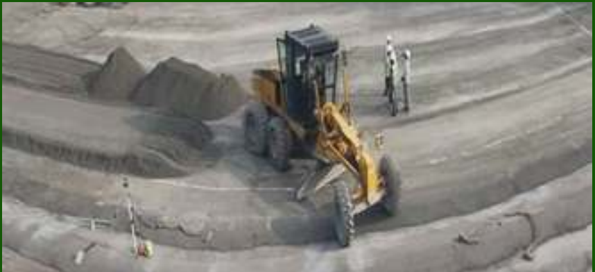
Low-carbon concrete mix strategies for the foundations of the Ayodhya Ram Mandir.
