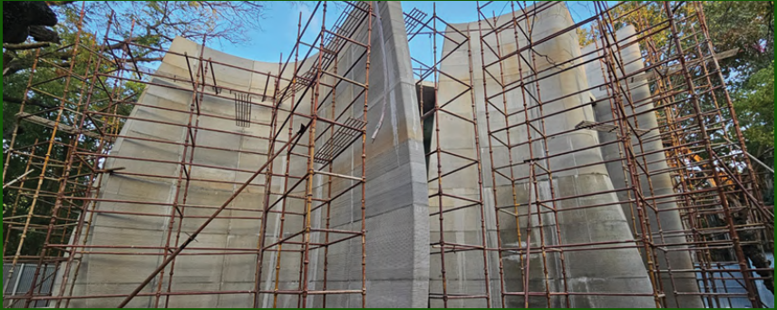
Construction of G+1 3D Printed Guest House on IIT Madras Campus
