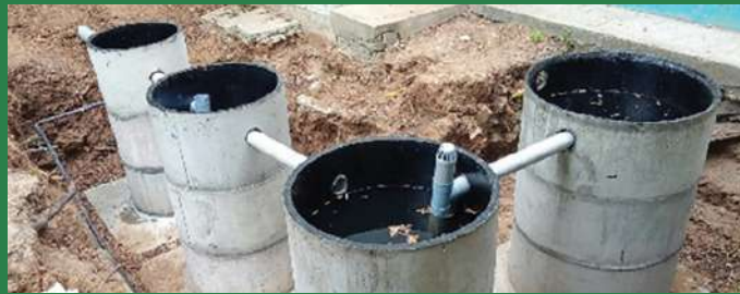
Textile Reinforced Concrete Precast Units
