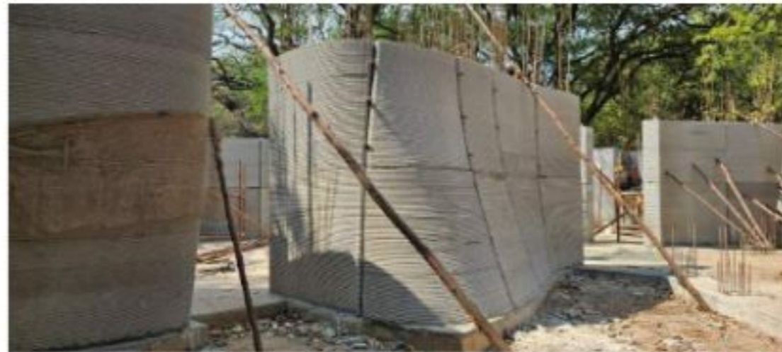
Guest house construction (3D concrete printing) IIT Madras, Chennai
