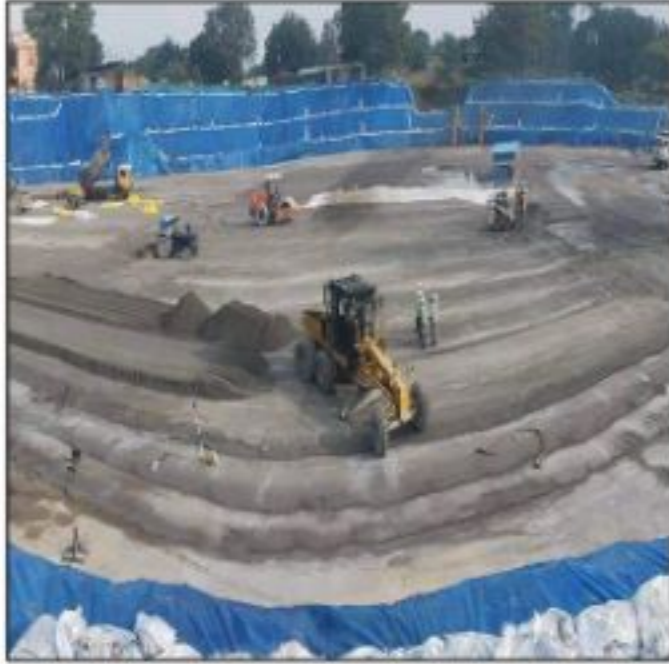
Concrete foundation (1000-year design life) Ayodhya
