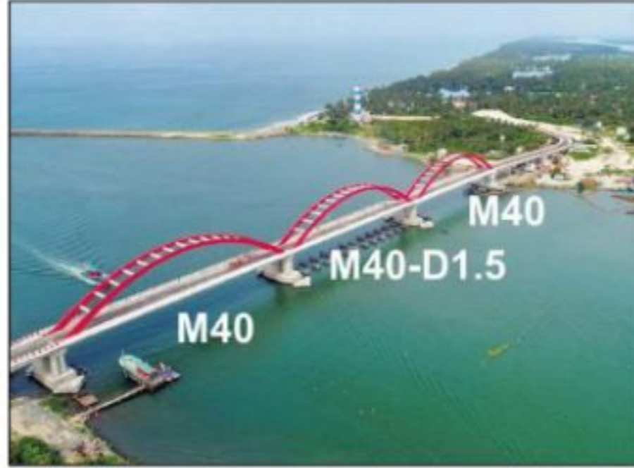
125 years service life Coastal Bridge, Kollam, Kerala
