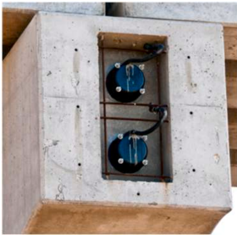
Fig. 1. Photo of a girder with permanent non-metallic anchorage caps [6].
