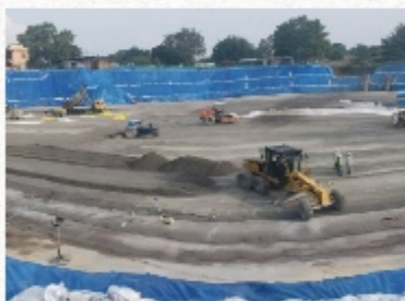
Low-carbon roller compacted concrete foundation with 1000-year design life, Ayodhya.
