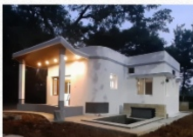
India's first 3D printed house (IITM-TVASTA initiative)
